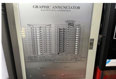
Fire Alarm Control Panel
